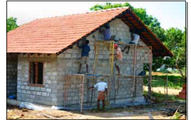
Workers working on a house
